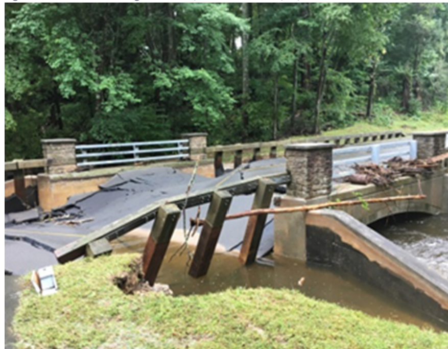
Figure 4.1 Washed Out Bridge in Chester, After Storm of 10/22/18
