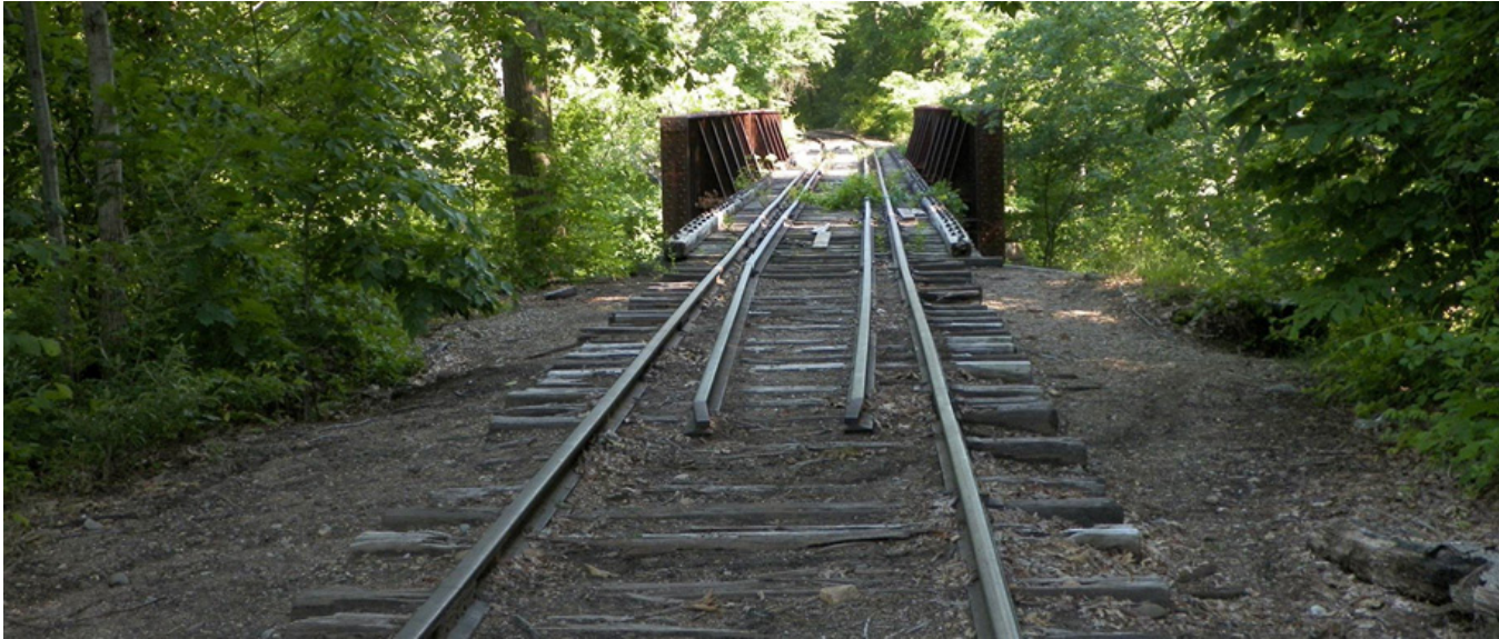
Figure 4.6 Valley Railroad State Park: Deteriorating track and vegetation on Higganum Cove bridge
