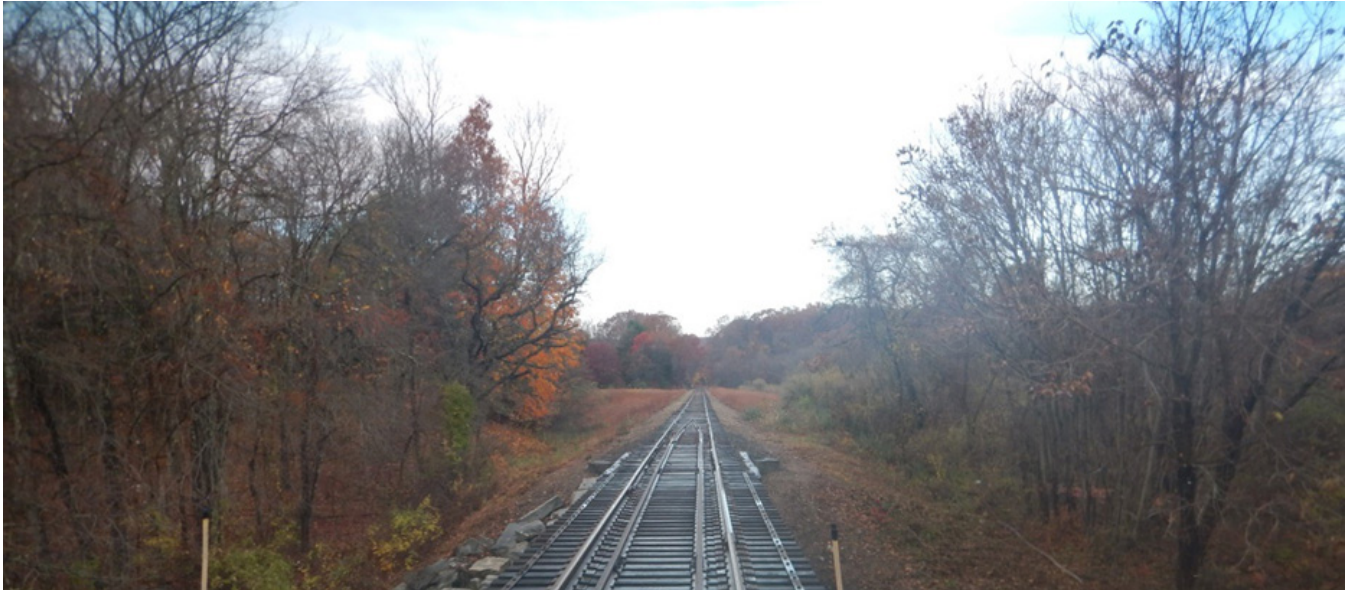
Figure 4.5 Valley Railroad State Park: Rail maintained south of Haddam
